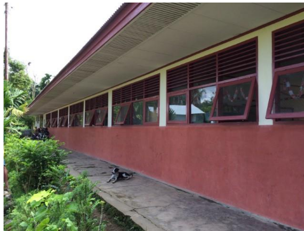
Figure 5 Large window openings are typical and present a weakness for the stability of the building for masonry shear wall construction
