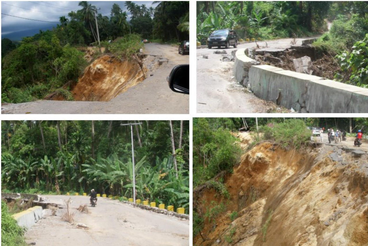
Figure 7 Roadway damage due to slope failures in Padang Alai (on the southern margins of Maninjau caldera, ~30 NNE of Padang city), from [7].
