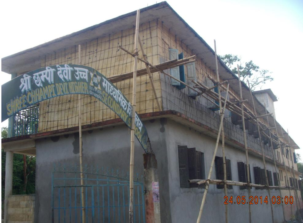
A two storied UCM-URM4 type of LBM school building strengthened using RC Jacketing technique. Note that the first story walls are already plastered (curing is ongoing) and the reinforcement mesh is being installed on the second story walls. (Photo from Nepal, Credit: Sunil Kumar Yadav, MoE, Nepal).
