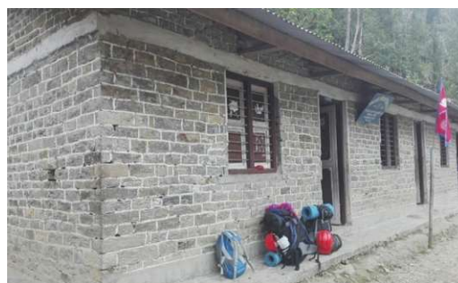
Illustration 2.11. Typical UCM-URM6 school building (Photo from Nepal, Copyright: The World Bank).
