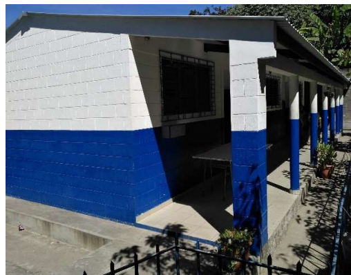
Illustration 2.14. Typical RM school building (Photo from El Salvador, Copyright: The World Bank).
