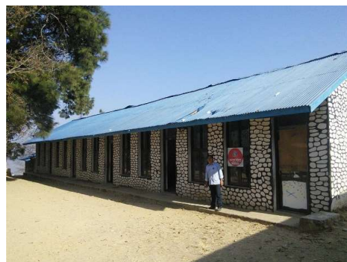
Illustration 2.10. Typical UCM-URM5 school building (Photo from Nepal, Copyright: The World Bank).
