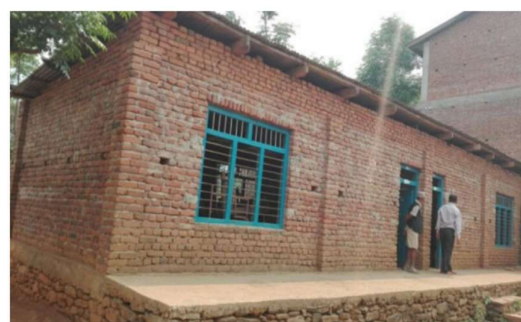
Illustration 2.12. Typical UCM-URM7 school building (Photo from Nepal, Copyright: The World Bank).
