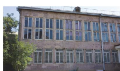
RC6: Precast RC frame with exterior
