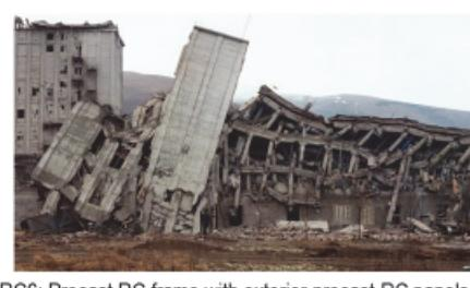
RC6: Precast RC frame with exterior precast RC panels
