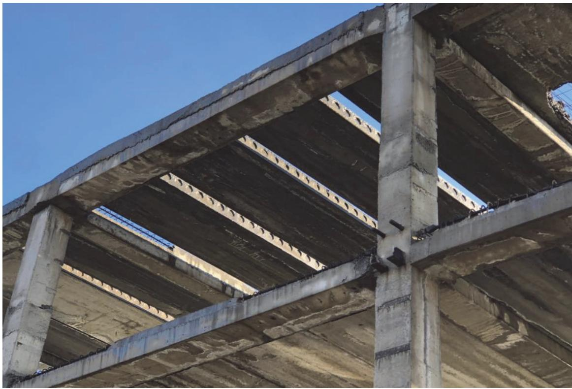
Figure 5-37 Beam-column connection in typical precast lateral-load-resisting system.
