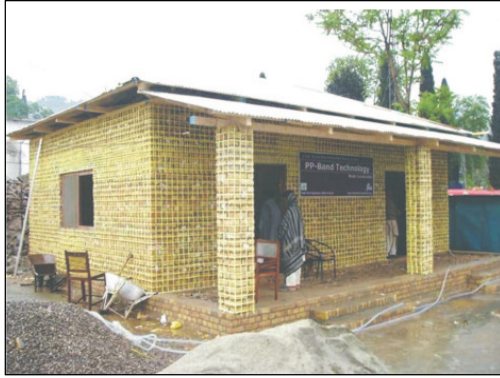
Retrofitted house in Pakistan using the PP Band meshing: Application of PP band (left) and building after plastering (right) (Reproduced from Macabuag et al. 2010)
